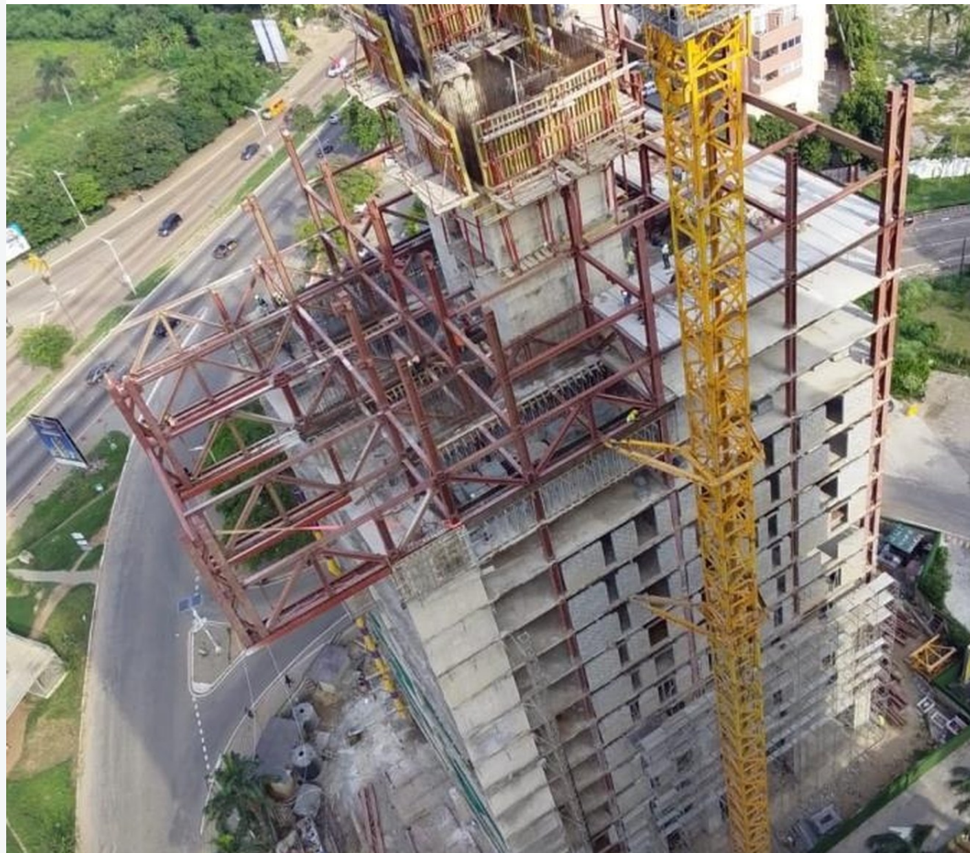
Reinforced-concrete core and advancing steel frame
